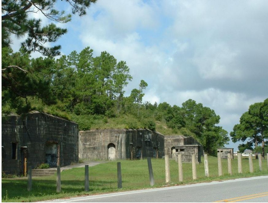
Figure 4-11: Batteries at Fort Morgan
